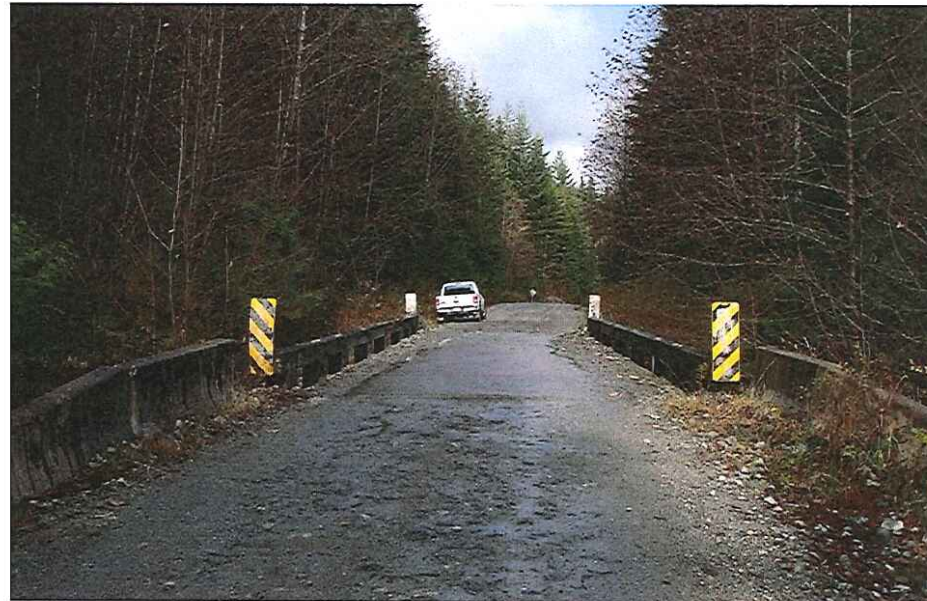
CK2096 Approach Right Bank
