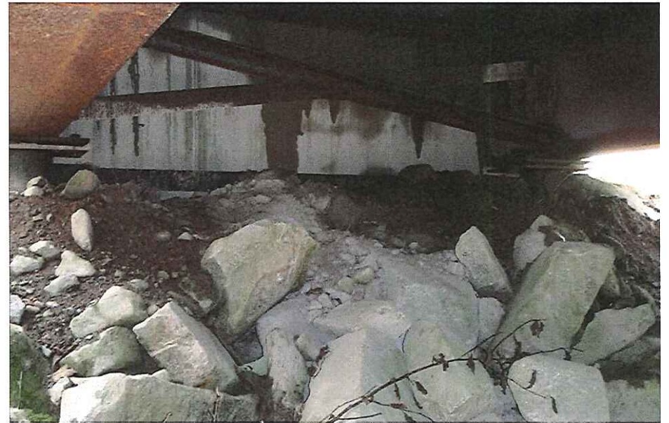
CK2096 Abutment Left Bank
