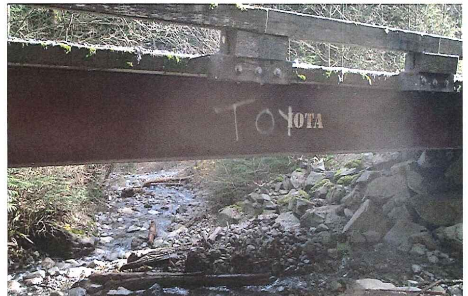
CK2096 Crossing Upstream
