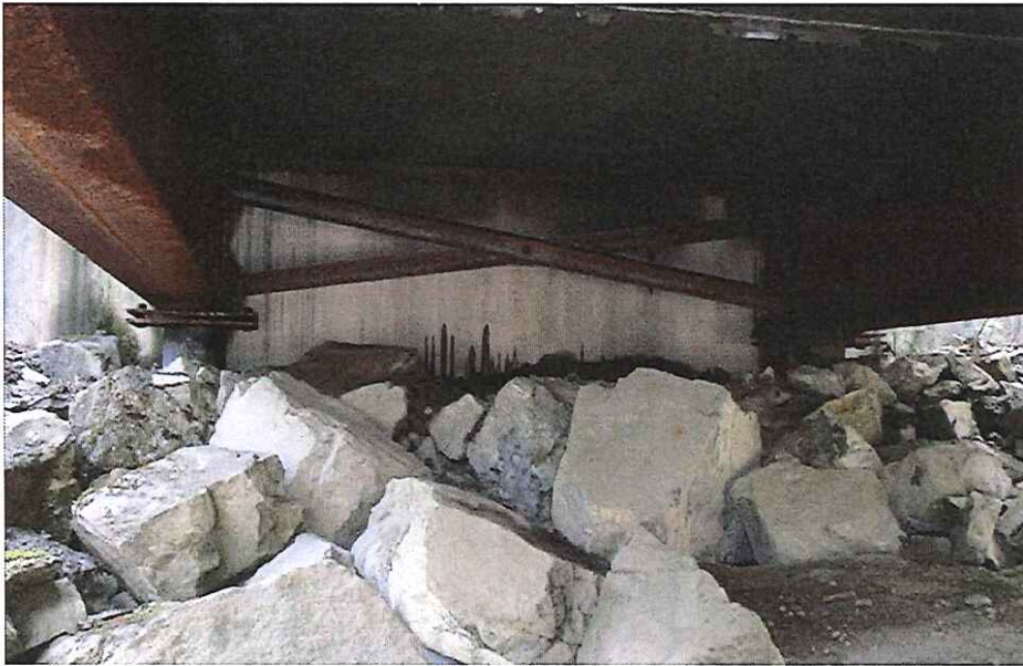
CK2096 Abutment Right Bank
